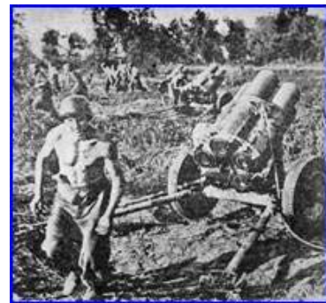
21cm Rocket Projector (Nebelwerfer). Range 10,000yds.
